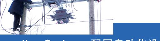
10Kv ZW20□−user demarcation circuit breaker 10Kv FZW28□—user demarcation load switch
